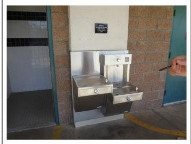
**Building 6** New hydration station, not built in compliance with accessibility guidelines.
